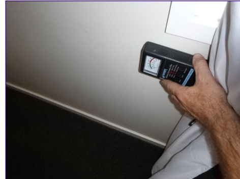
Dry at the time of the inspection.
