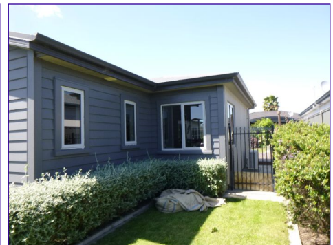
West facing wall
