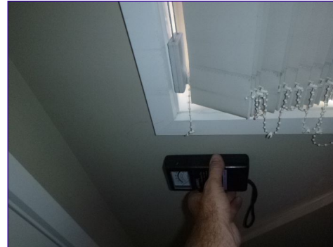
Dry at the time of the inspection.
