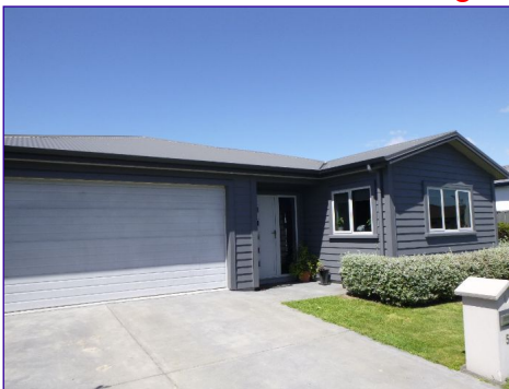
North facing wall
