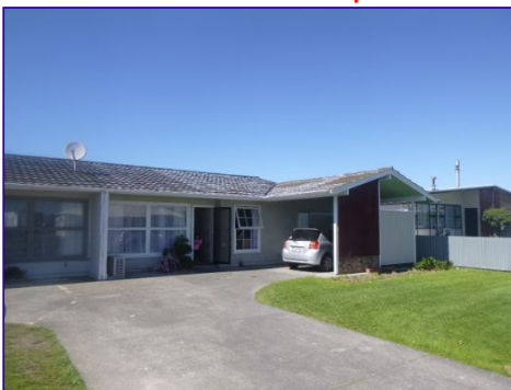
North West wall
