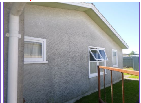
South West wall
